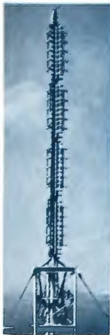
Directional VHF-TV Transmitting Antenna
